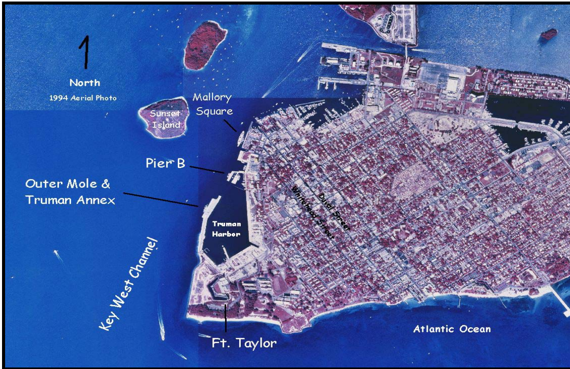
FIGURE 3.A.14. 1994 AERIAL VIEW OF KEY WEST CHANNEL AND HARBOR WITH CRUISE SHIP BERTHS NOTED.
